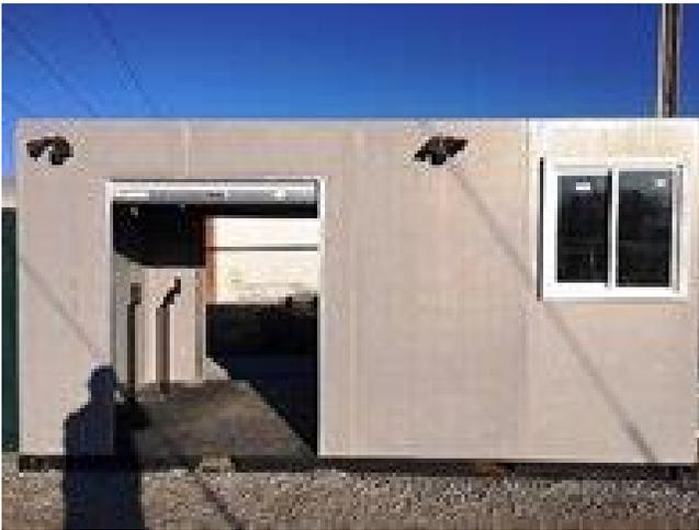
The building itself is weather-proof fiberglass, constructed in 2' sections. This base model is 8' deep by 18' long with an 8' high ceiling. The size is customizable in 2' increments to fit the end user's needs.
