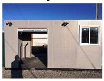
The building itself is weather-proof fiberglass, constructed in 2' sections. This base model is 8' deep by 18' long with an 8' high ceiling. The size is customizable in 2' increments to fit the end user's needs.
